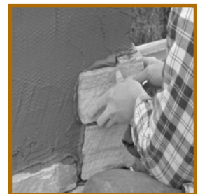
← PHOTO #3 - Application of mortar onto Natural Thinstone Veneer.
