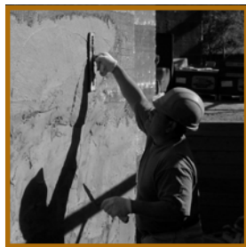
PHOTO #2 - Application of scratch coat to surface of exterior wall.
