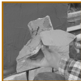
← PHOTO #3 - Application of mortar onto Natural Thinstone Veneer.
